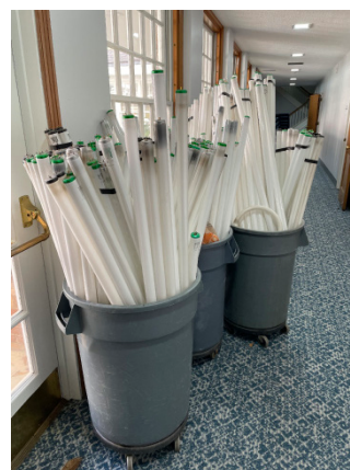
Flourescent lightbulbs that were replaced by LED bulbs
