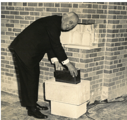
Payne Midyette, Chair of the Building Committee, at the laying of the cornerstone in February 1964.
