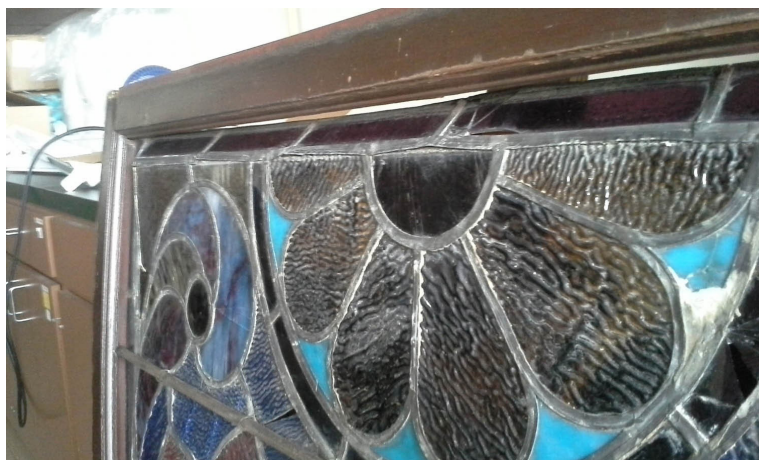
Bent bottom of window
