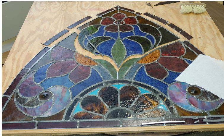
Separating top from bottom sections
