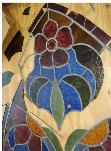
Repairing the top portion of the window
